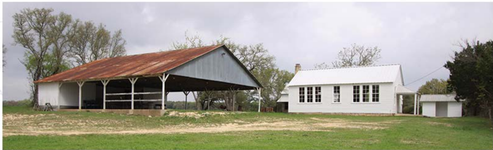
In his book "A Journey Through Texas," Frederick Law Olmsted observed in Rheingold Common School/Community Center. The stage and pavilion (left) was built 1936; the second schoolhouse (right) was built 1881. - photo by Ben Shacklette, AIA
