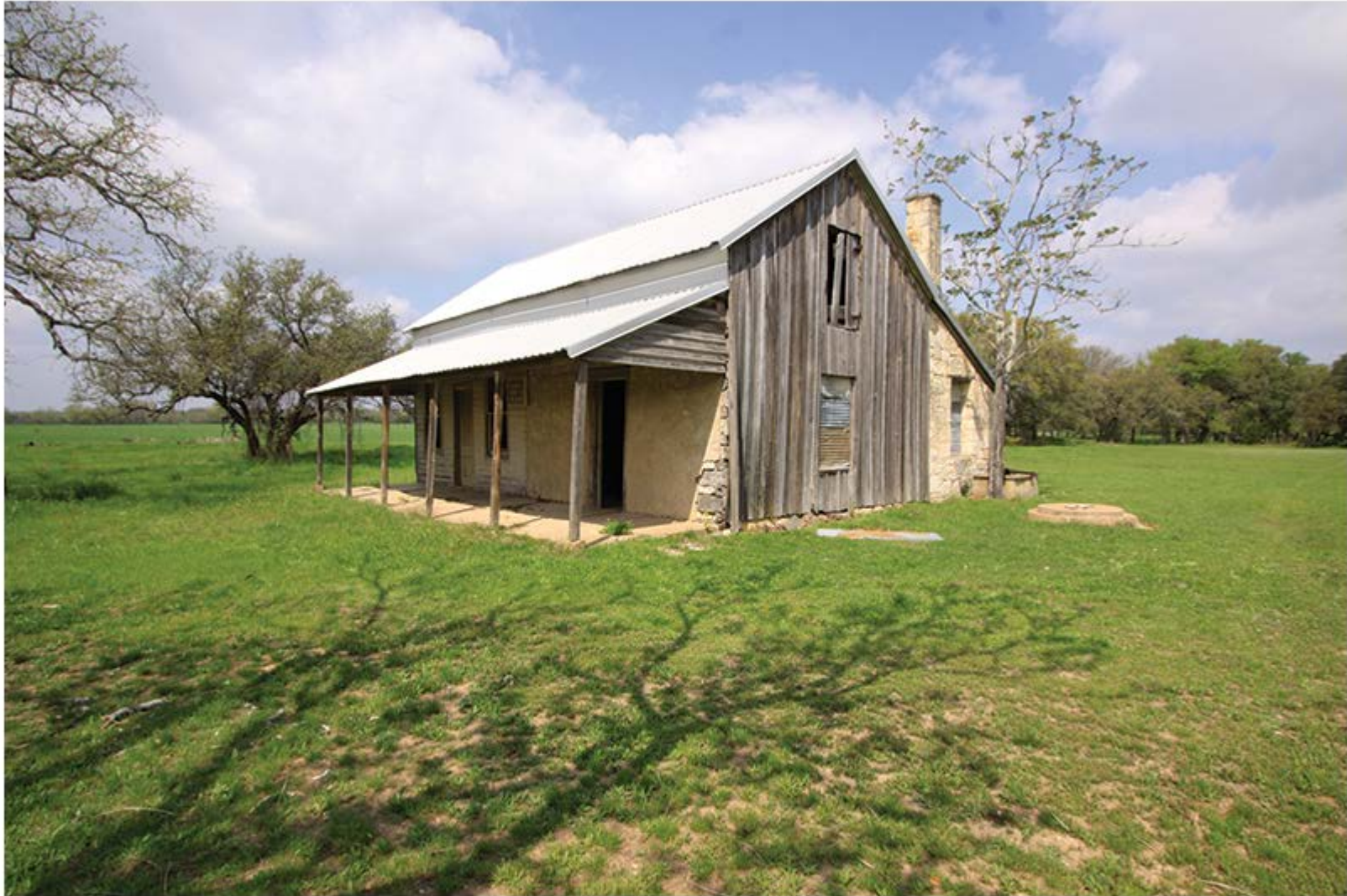
citizens instigated the signing of Texas Senate Bill 116 in 2002, which changed Texas law to Rheingold Common School/Community Center. The log-framed limestone schoolhouse was built in 1878 and served as a teacherage after 1881. - photo by Ben Shacklette, AIA
