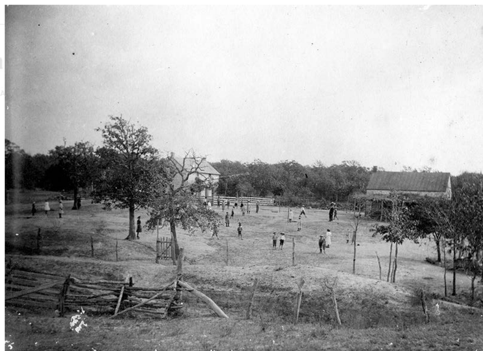
no cost. Today, The Friends of Gillespie County Country Schools oversees 12 historic Palo Alto Common School, c. 1900. The log school with a brush arbor porch (right) was built in 1869 and converted to a teacherage when the limestone schoolhouse (left) was erected in 1883. In 1934, enrollment peaked at 65 pupils taught by two teachers covering grades one through nine. The school finally closed in 1946. - photo courtesy Gillespie County Historical Society, Fredericksburg, Texas
