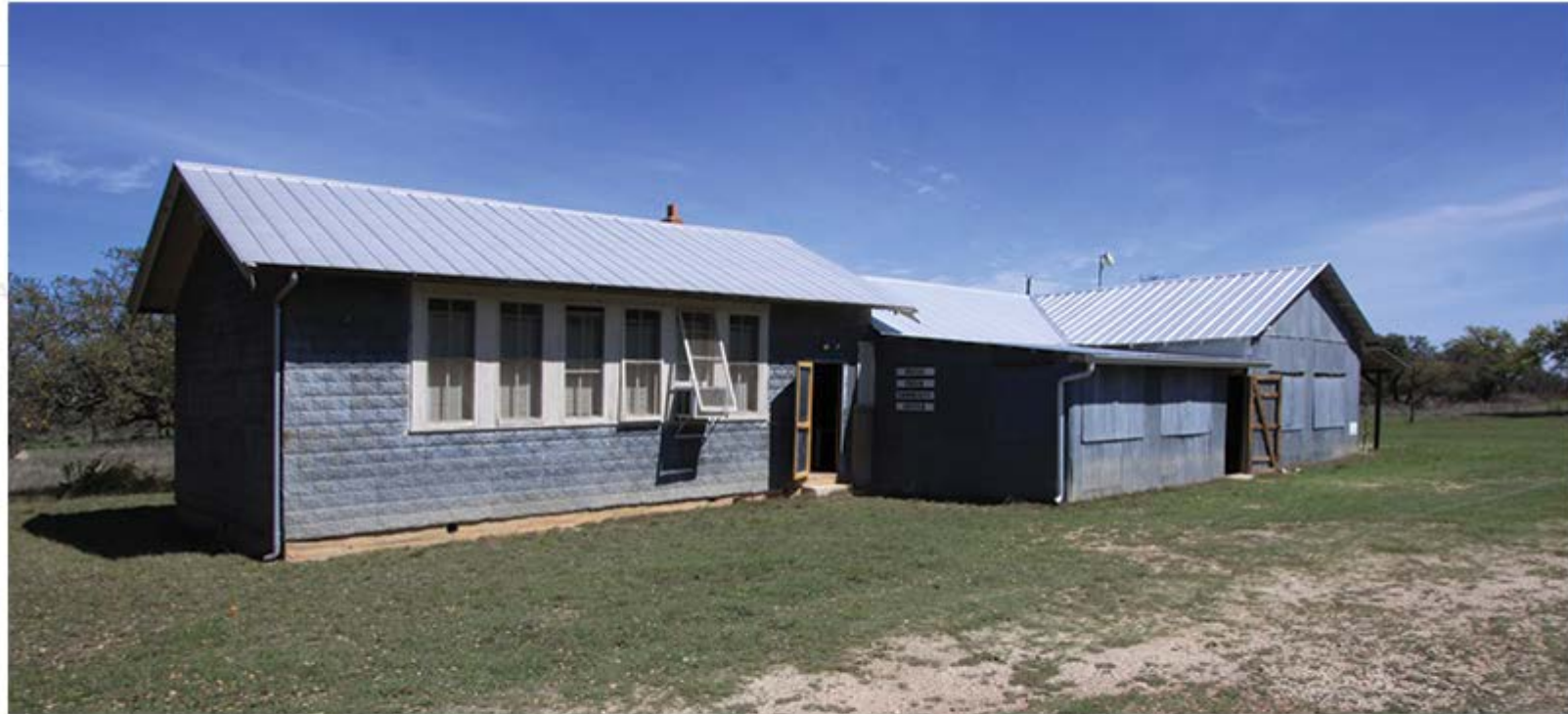
Pecan Creek Common School/Community Center. The schoolhouse (left) was constructed in 1916 using wood framing with embossed tin siding. The attached pavilion (right) was constructed between 1936 and 1940 using timber framing with corrugated steel siding. - photo by Ben Shacklette, AIA
